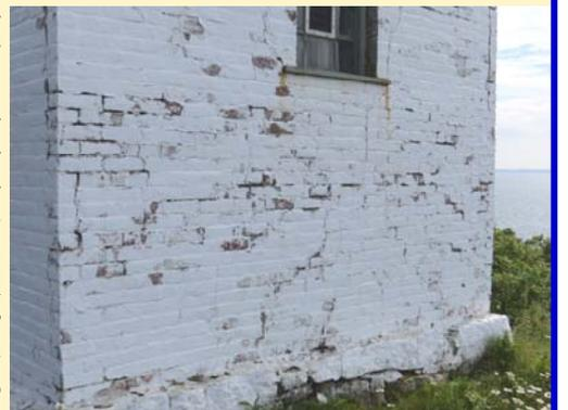
**Closer scrutiny reveals the extensive deterioration of the brick** *Elke Dorr*
